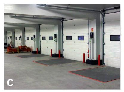
To comply with the new walking-working surface regulations, an employer is required to either equip their dock equipment with run-off guards or demonstrate that no risk for transfer vehicles to run-off the dockboard edge exists. LODEM recommends that employers utilize dockboards or dock levelers that comply with ANSI MH30.1 and ANSI MH30.2, respectively. Furthermore, when dock levelers without run-off guards are used,
